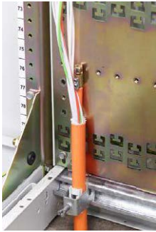
Cable attachment plate with C-profile
