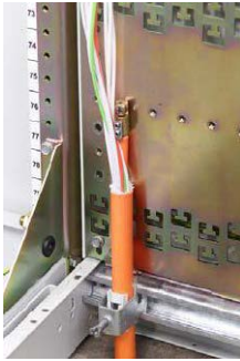
Cable attachment plate with C-profile
