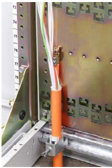
Cable attachment plate with C-profile
