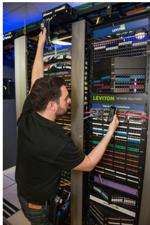
Reading FiberChek probe results on a smartphone
