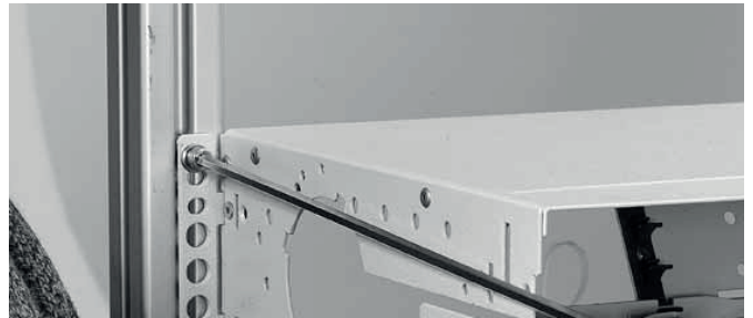
1.1.2 Mount the shelf using the Screwdriver.
